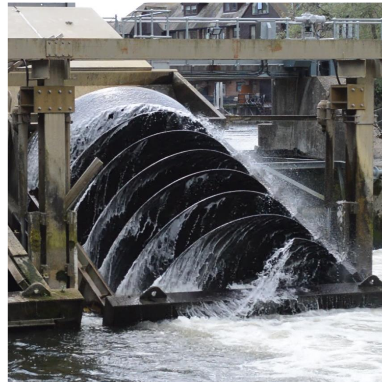
Windsor Castle Powerplant Romney Lock, Windsor and Maidenhead, UK
