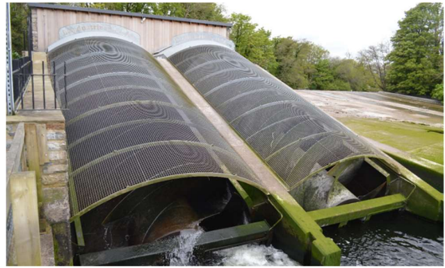
Figure 2: the "sloshing phenomenon" was observed and noted in a field study the author's conducted on an Archimedes screw generator powerplant in Totnes, United Kingdom.
