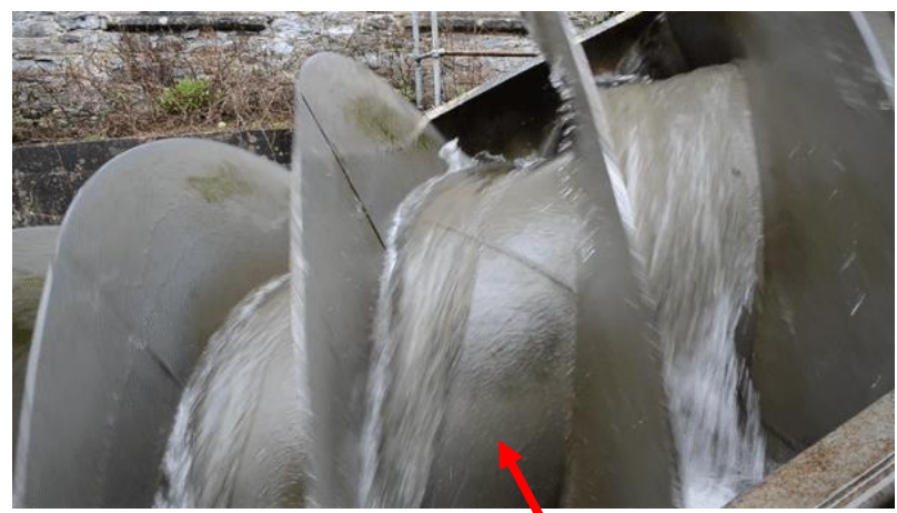
Overflow Leakage
