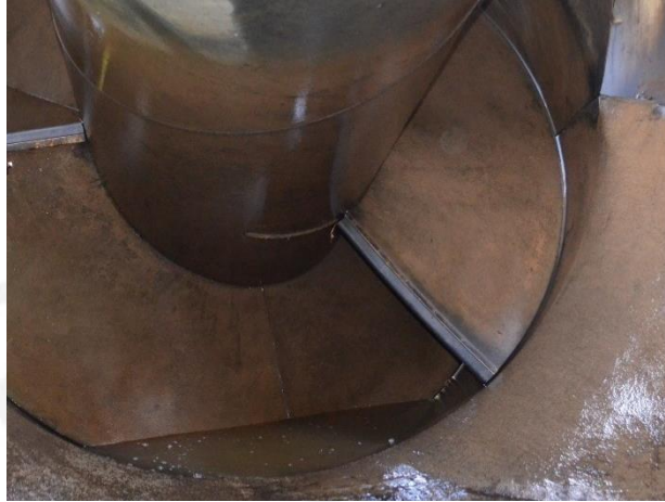
183 Figure 3: View inside the forebay of the Ruswarp Hydro ASG. Blade leading edges have rubberized bumpers to minimize 184 impact damage to aquatic fauna.
