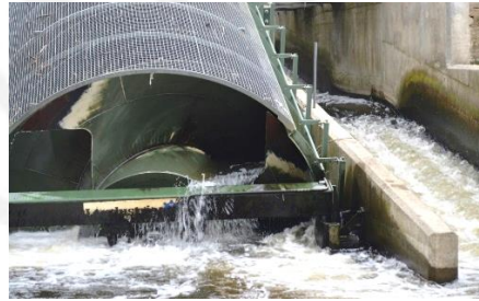
420 Figure 5: Modified blade ends at the Goldsborough ASG outlet.
