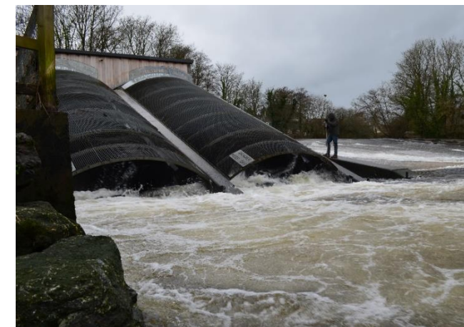
Lubitz, W. D. (2019), Totnes Hydro Powerplant.
