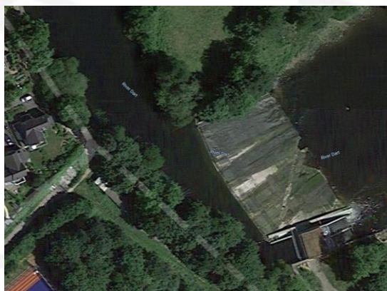
318 Figure 11: Totnes power plant has a short inlet and significant outlet water level variation due to impacts of ocean tides. 319 North is upward. The plant is at lower right on the south end of the weir. Flow is from left to right. 320
