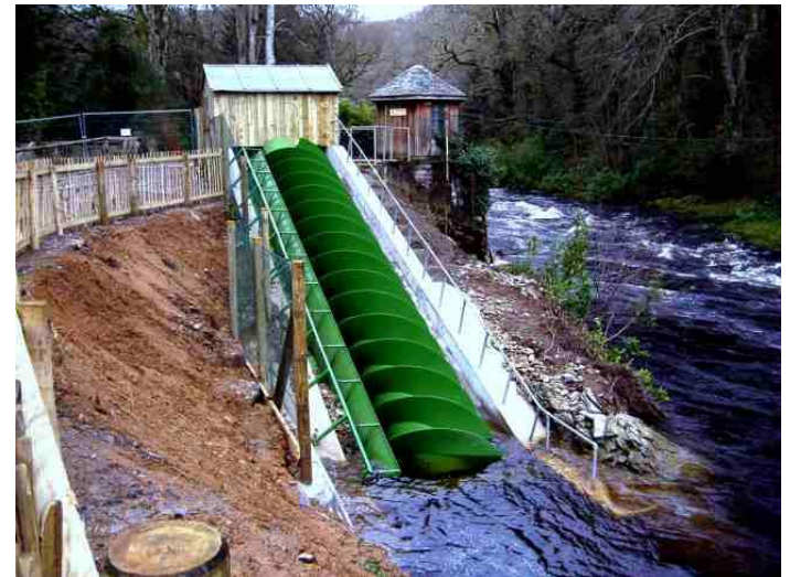
Archimedes screw generator installation (Western Renewable Energy, 2019).
